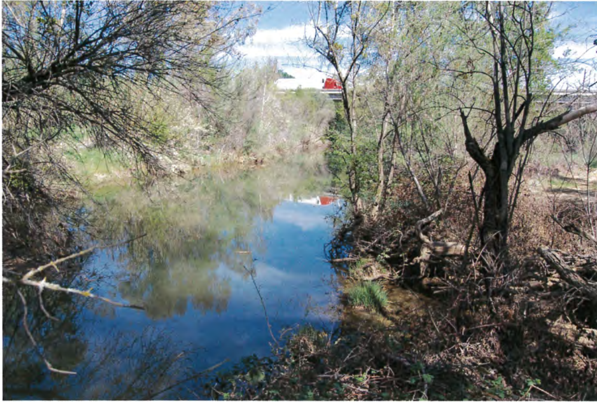
Photo 3 – Looking east at the over-widened low-flow channel and the I-505 bridge in the background. Phase 2 will narrow this segment of channel.
